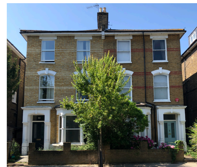
Fig 5.6 Three storey semi-detached property, Wilberforce Road
