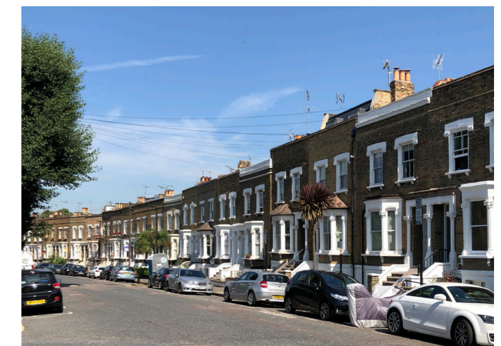
Fig 5.12 Terraced housing, Mountgrove Road
