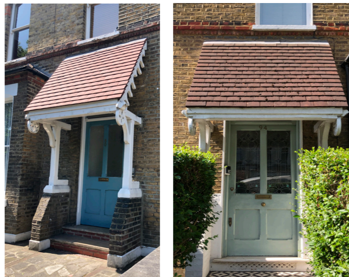
Fig. 5.2 & Fig. 5.3 Distinctive porches with original four panelled doors
