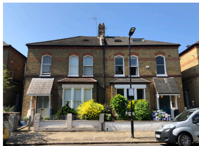
Fig 5.1 Finsbury Park Road
